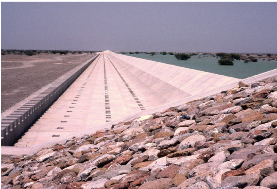
(b) Large recharge dam in the Batinah Plain, Oman [Photo: Jac van der Gun]. Flood water is retained by the dam and is subsequently released in a controlled way to recharge the aquifer zone downstream.
