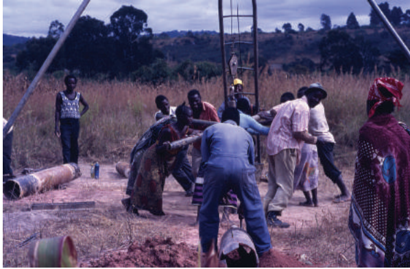
(a) Villagers drilling jointly by hand a shallow well in weathered basement rock, for community drinking water supply in Tanzania.
