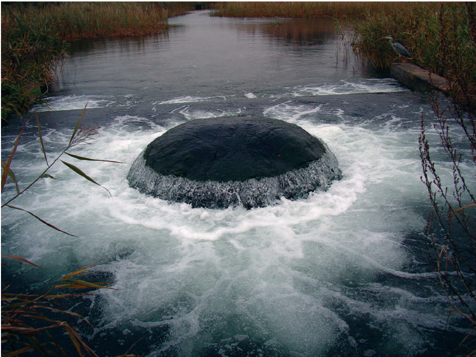
Figure 7.8 Open recharge canal in the dune area of The Netherlands, supplied by a surface water transport pipeline. [Photo: PWN].
