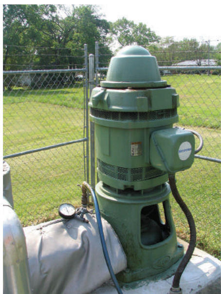
(a) Public water supply well with electrically powered line shaft turbine pump, USA [Photo: USGS].
