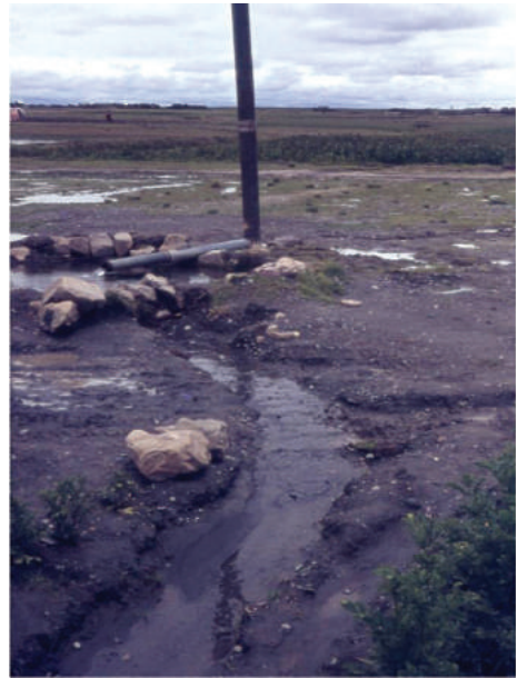
Figure 4.15 Artesian well on the Bolivian Altiplano. [Photo: Jac van der Gun]. The casing extends several metres above ground surface to ensure that no groundwater is spilt after the horizontal discharge pipe is closed.
